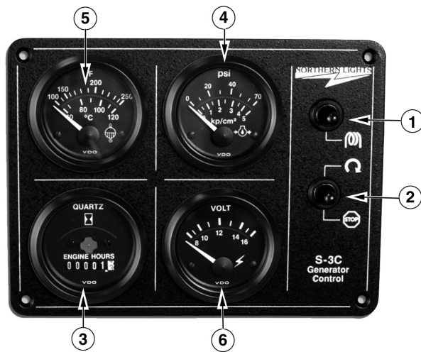
Figure 3-B: Series 3 Generator Control Panel
