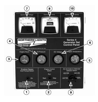
Figure 3-C: Series 4 Generator Control Panel
